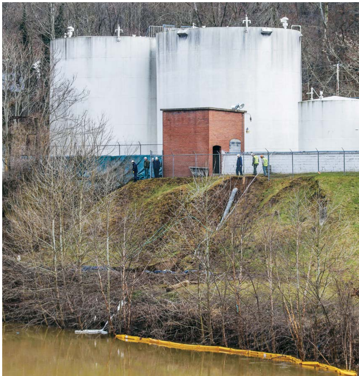
Potentially dangerous chemicals that spilled from these storage tanks on the Elk River outside Charleston, WV, affected the drinking water of 300,000 people. Yet due to a lack of regulation, virtually no data were available to health officials who dealt with the tragedy.
