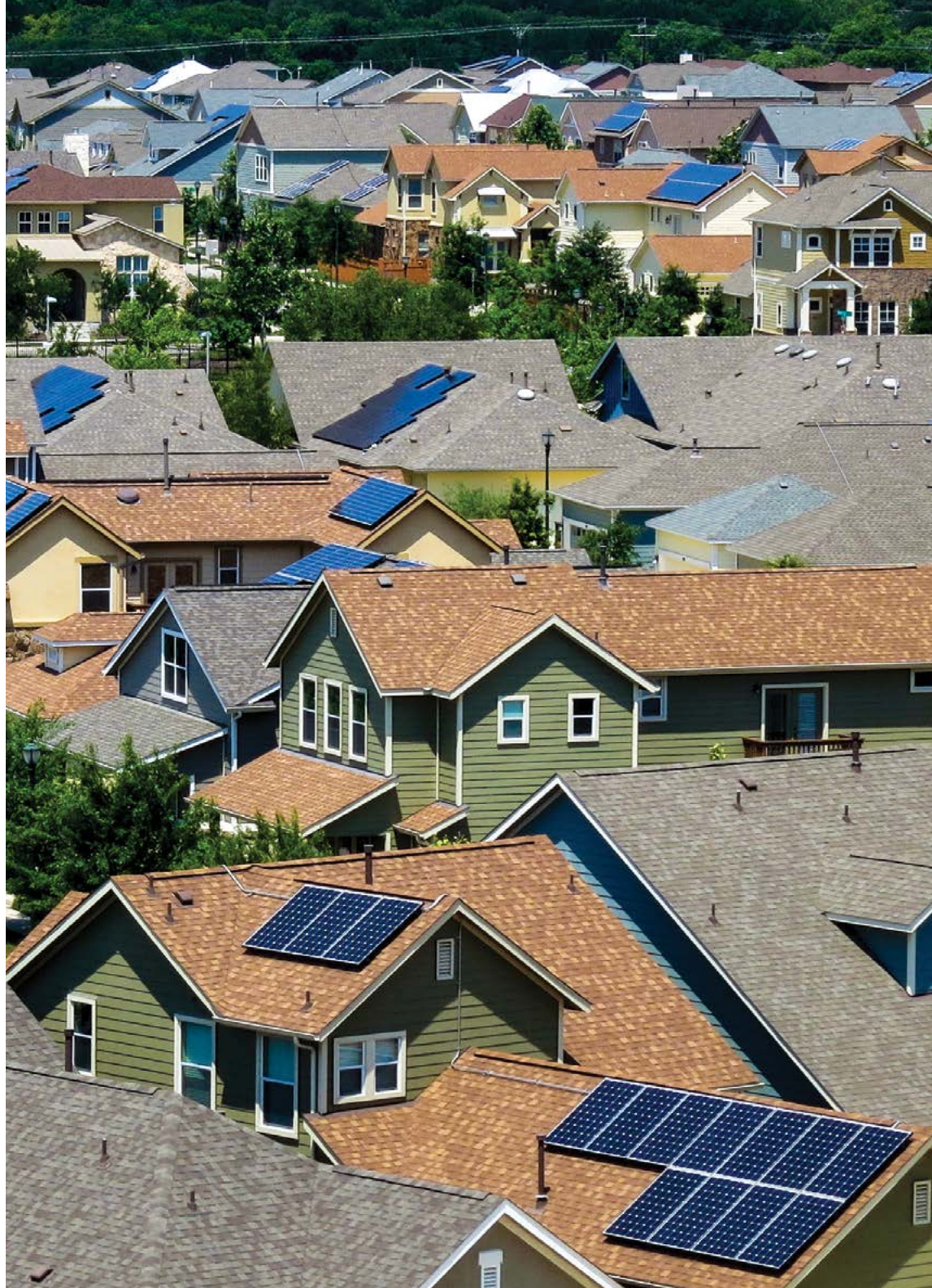
EDF co-founded Pecan Street Inc., in Austin, TX. Participating homeowners save money, and their homes use 38% less electricity on average for cooling, per square foot, than conventional houses.
